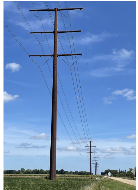
Example of double-circuit 345-kV structure.
