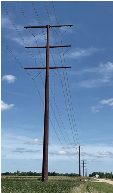
Example of double-circuit 345-kV structure.
